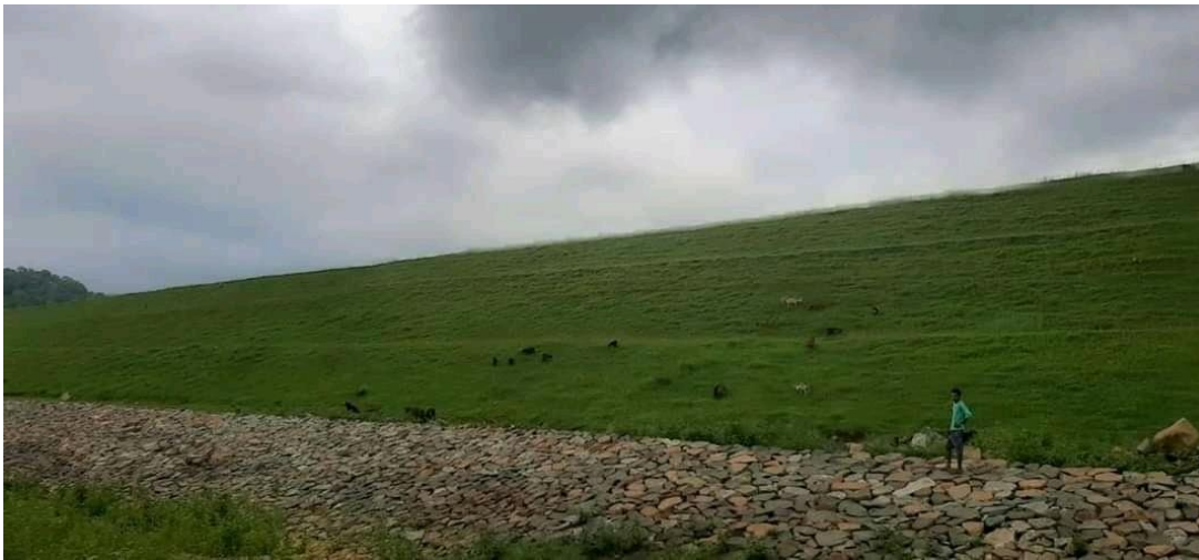
Deo Earthdam work
