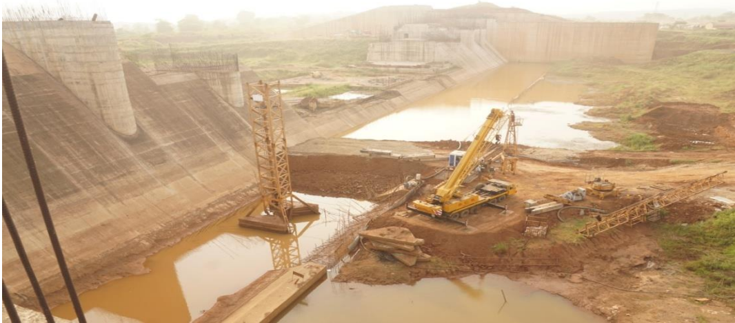
kanpur Spillway work
