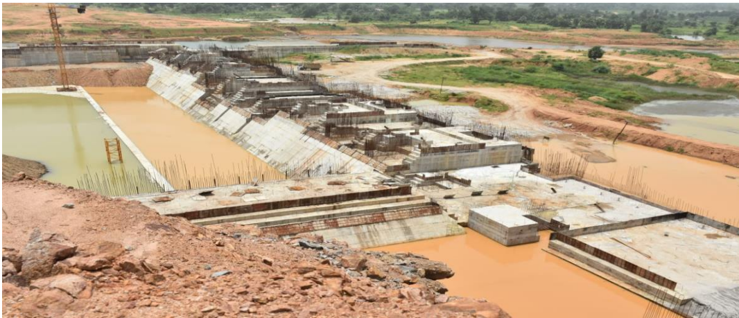
Lower suktel Spillway work
