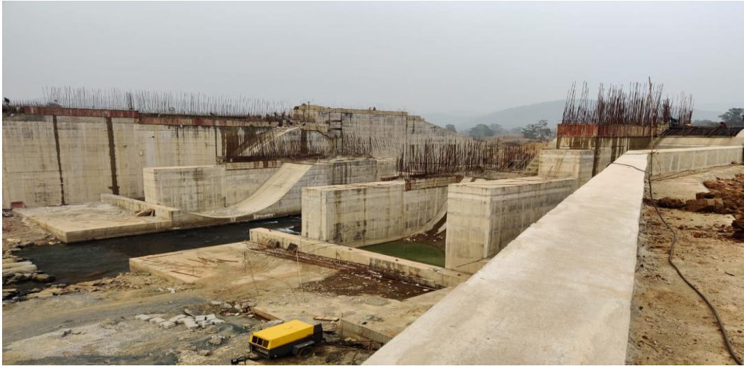
Deo Spillway work
